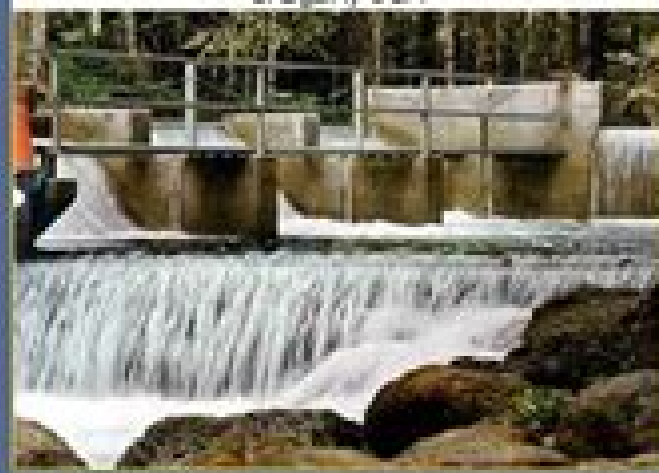
4.3-MW Run-of-River Hydro Project, Oregon, USA
